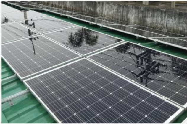
◀ Thailand (1) Installed Loop solar panel on the parking rooftop.
